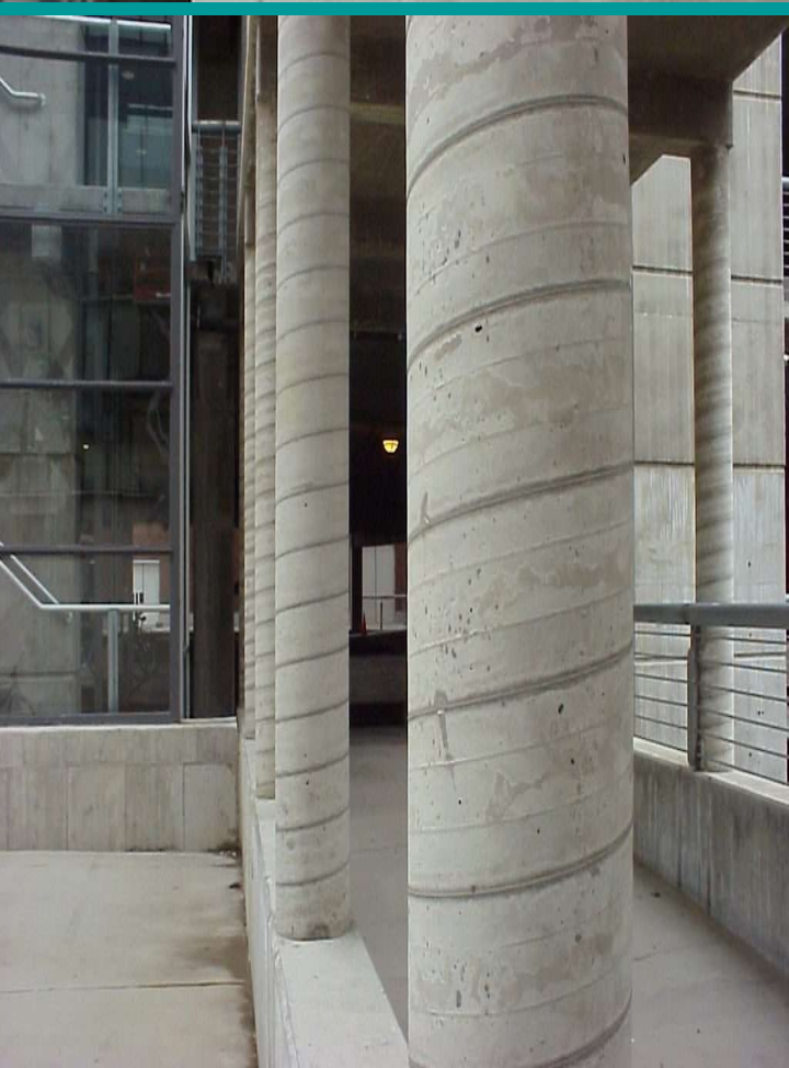
Stripped Column Note the spiral formwork marking
