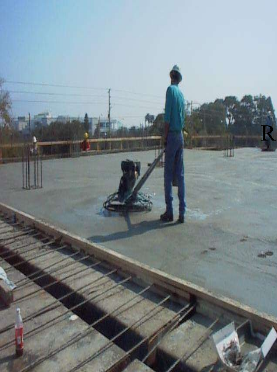
Finishing Rotary Power Trowel (Rider - Double Blade)
