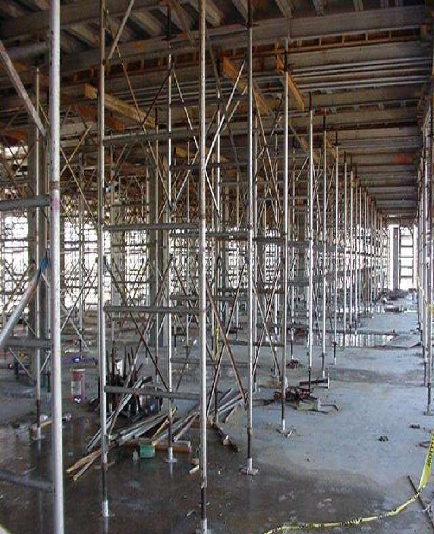
Shoring Support System (Scaffolding)
