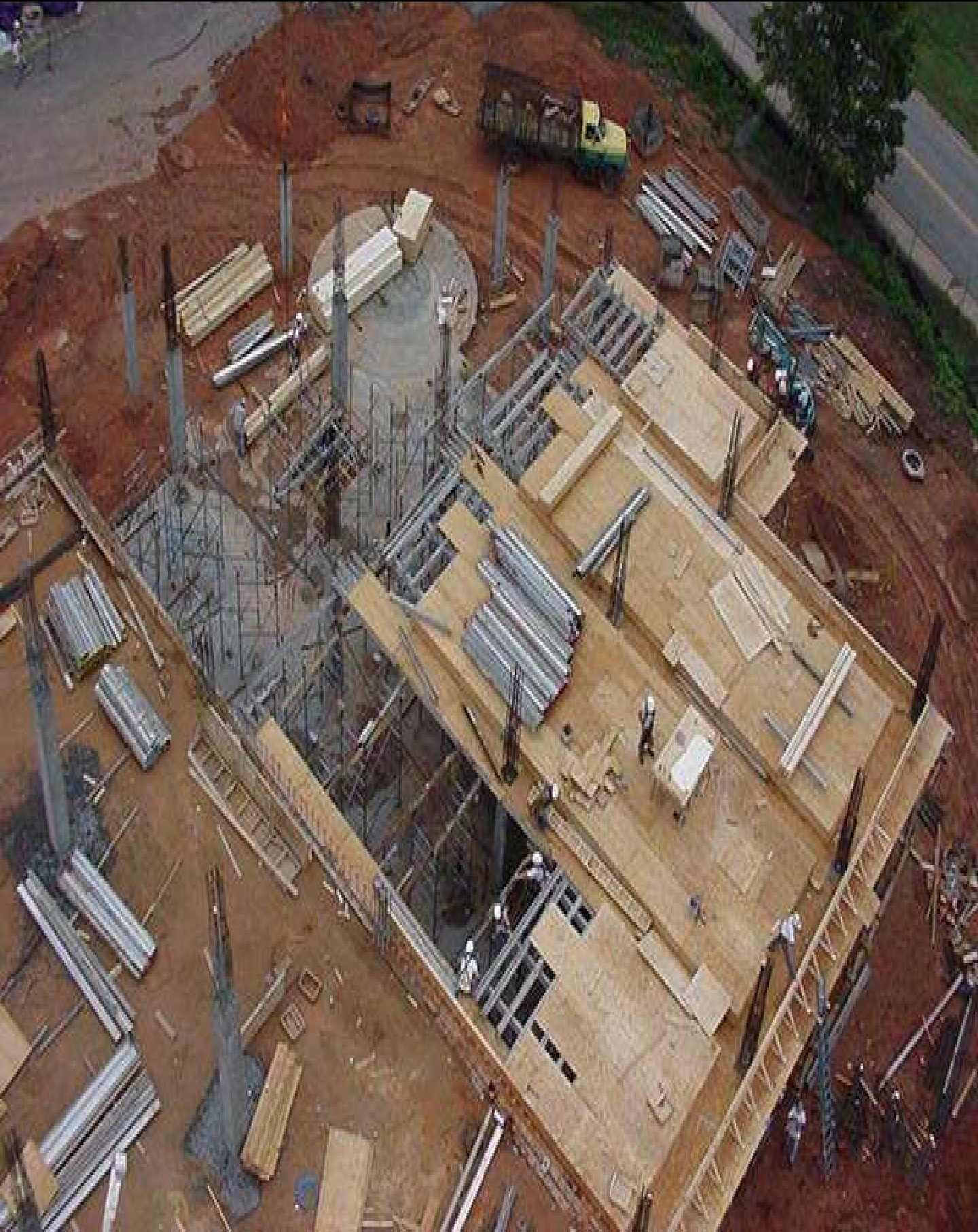
Wood Decking and Beam Sides Erected on a Portion
