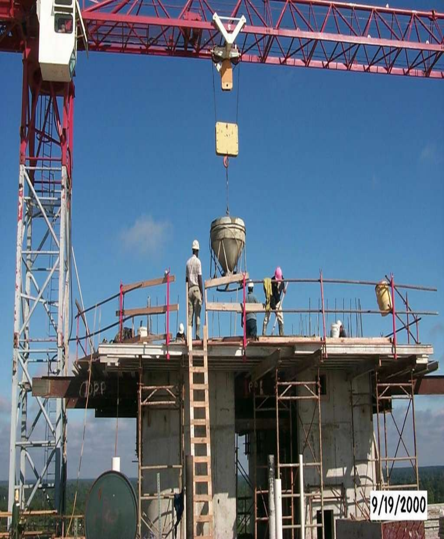
Placement of a Wall with a Crane & Concrete Bucket
