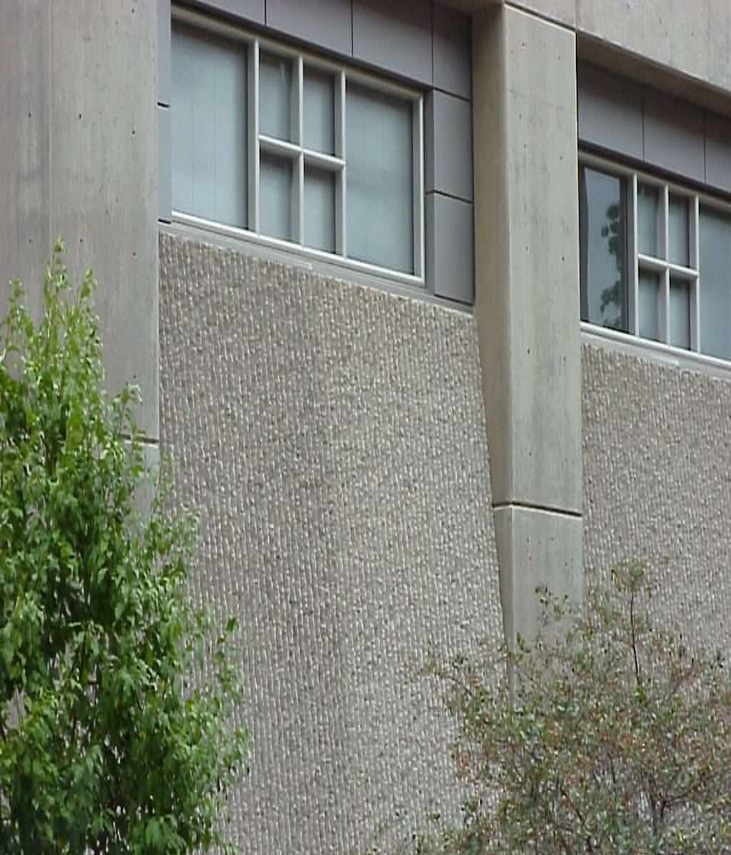
Architectural Concrete with “Bushhammered” Finish
