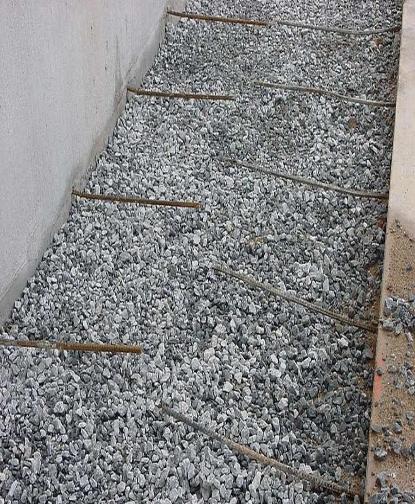
ade prepared for panel structural connection to Slab-on-
