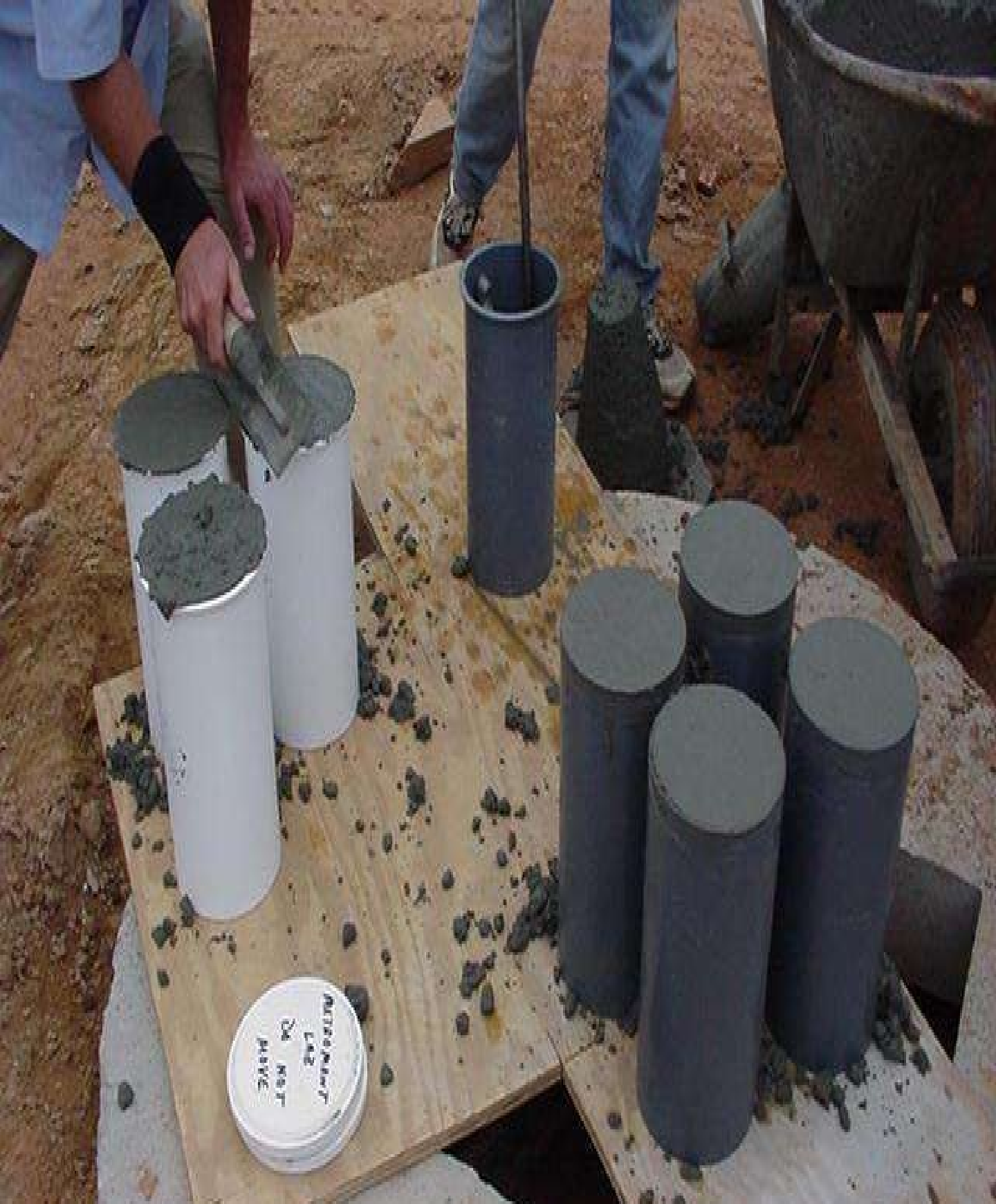
Test Cylinders Filled with a Sampling of the Concrete Mix
