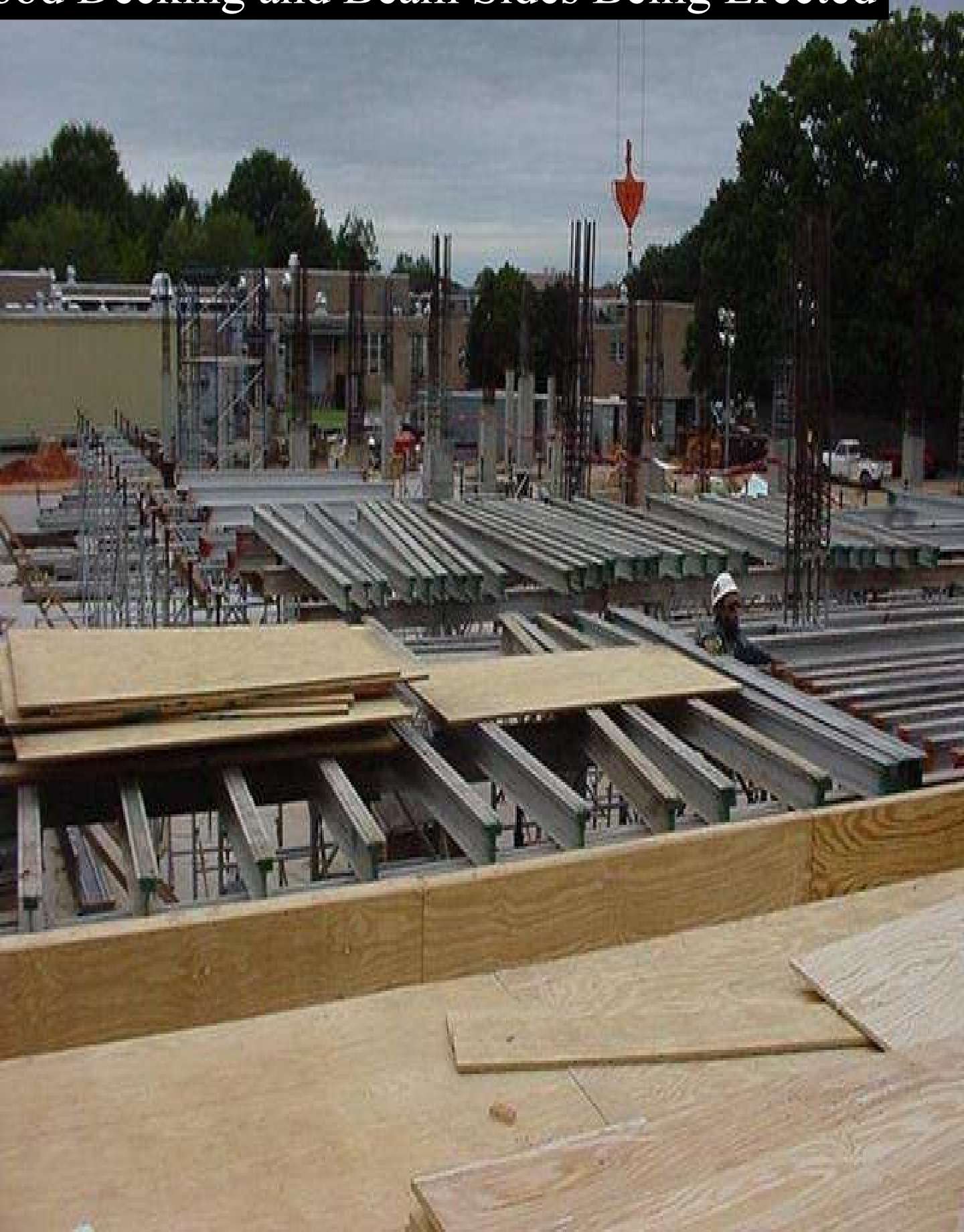
ood Decking and Beam Sides Being Erected
