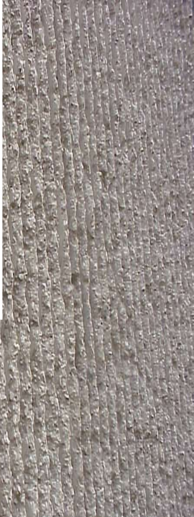
Architectural Concrete with “Bushhammered” Finish
