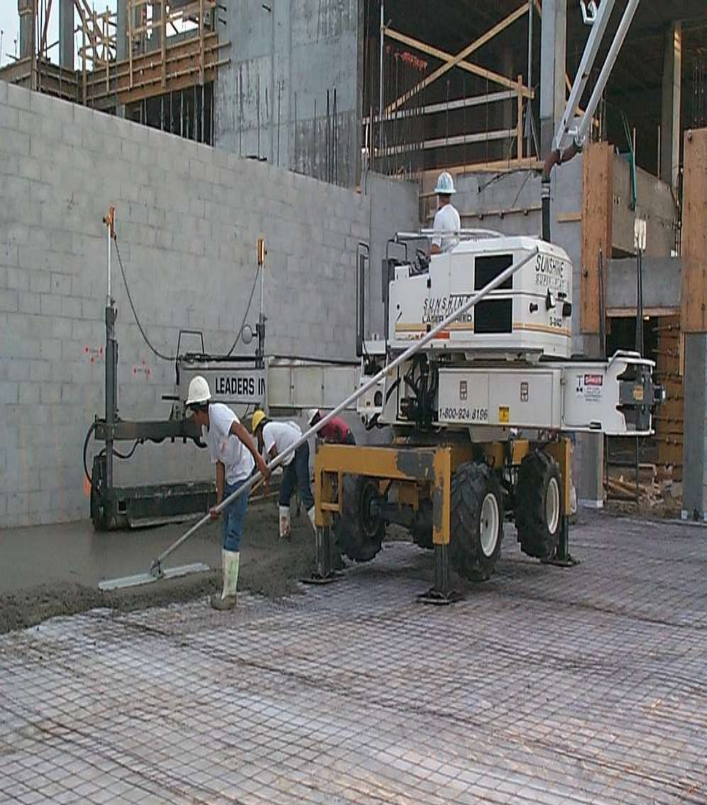
Laser-screed Often used for 'superflat' floors
