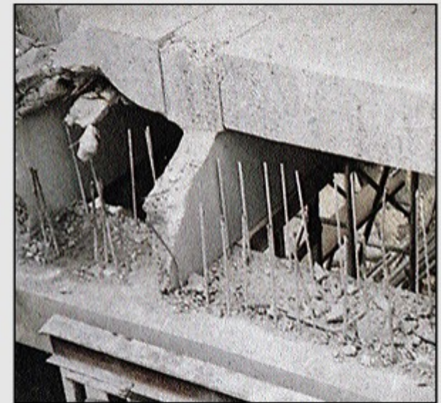
Photo A. Sections of this precast, prestressed double tee unit were shored, sawed and lifted out.
