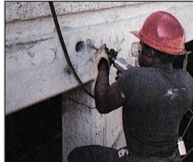
Photo B. Detensioning the tendon releases its force and allows safe removal of post-tensioned concrete sections. Here a laborer is chipping grout out of an anchorage pocket to allow access for a hydraulic
