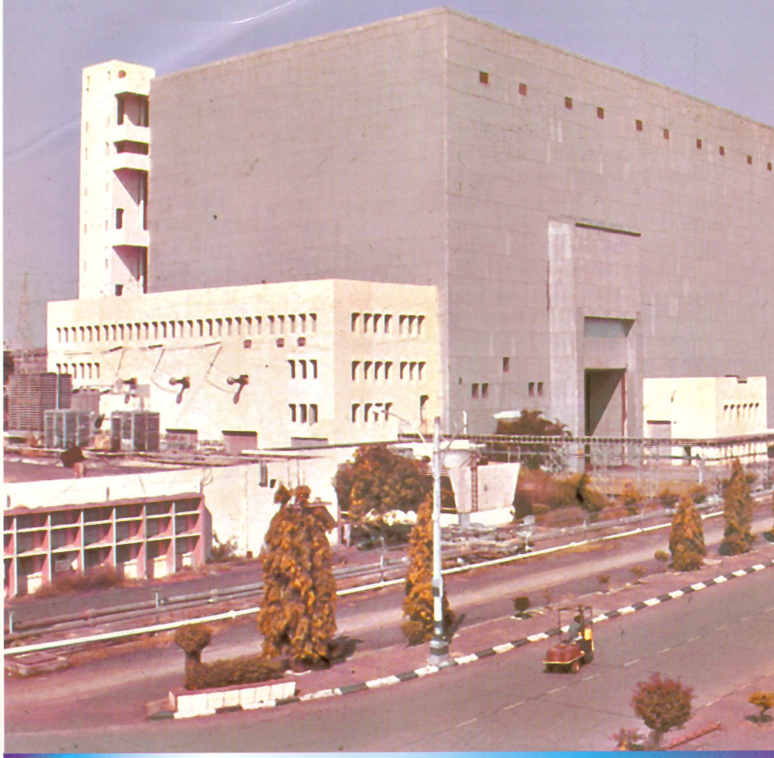
View of Ultra High Voltage Test Lab
