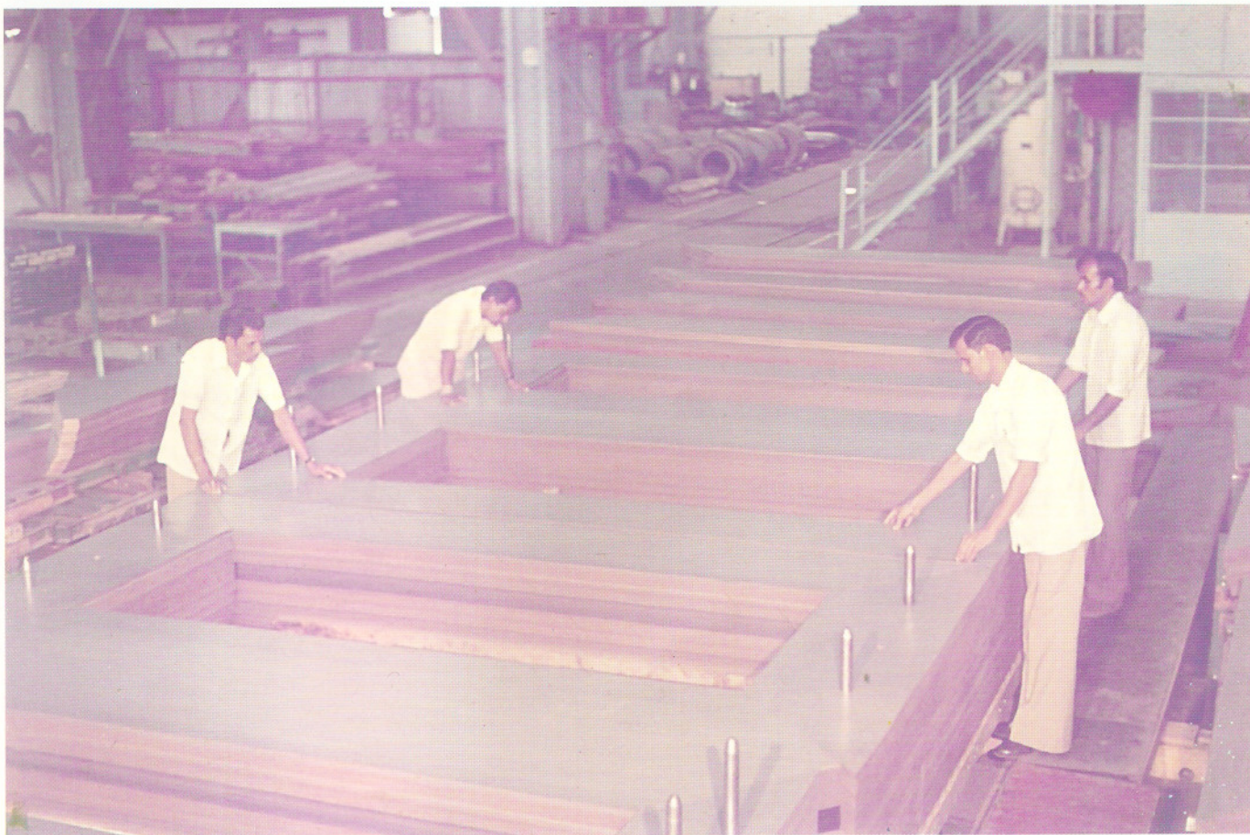
Core of a 240 MVA 15.75/420 kV Generator transformer under construction
