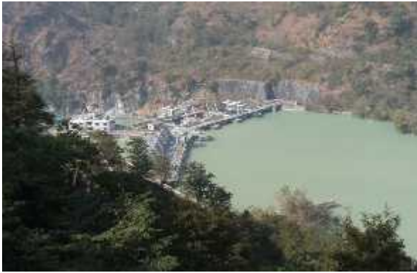
Dam site of Kaligandaki Hydropower Project
