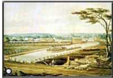
Figure 3-3 View of Erie Canal by John William Hill, 1829. Packet boat on the Erie Canal
