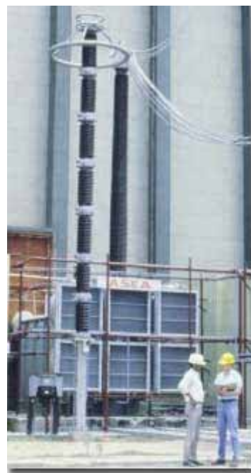
Oil-immersed smoothing reactor in the Rihand - Dehli HVDC transmission
