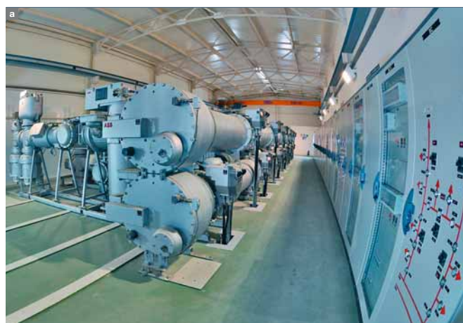
3 Typical substation with GIS of ELK-04-type in Spain (Mallorca) a and replacement of AIS by GIS of ELK-04-type in the United States (California) b
