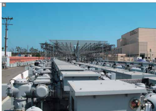
3 Typical substation with GIS of ELK-04-type in Spain (Mallorca) a and replacement of AIS by GIS of ELK-04-type in the United States (California) b
