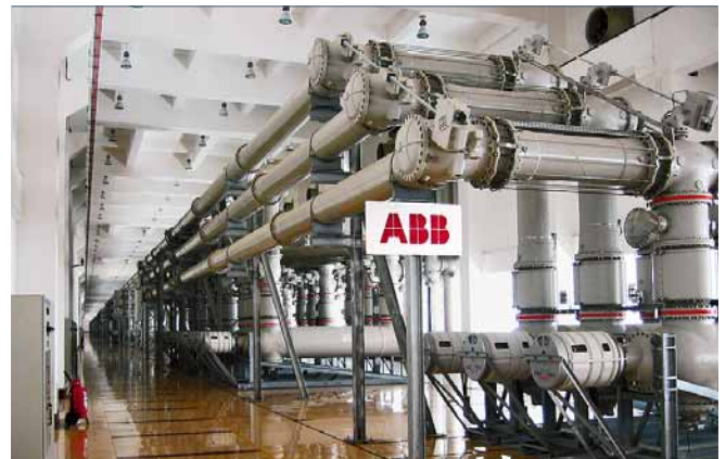
5 A 550 kV substation with GIS (rated at 550 kV, 63 kA, 4,000 A) installed within the dam at Three Gorges hydroelectric power plant in China
